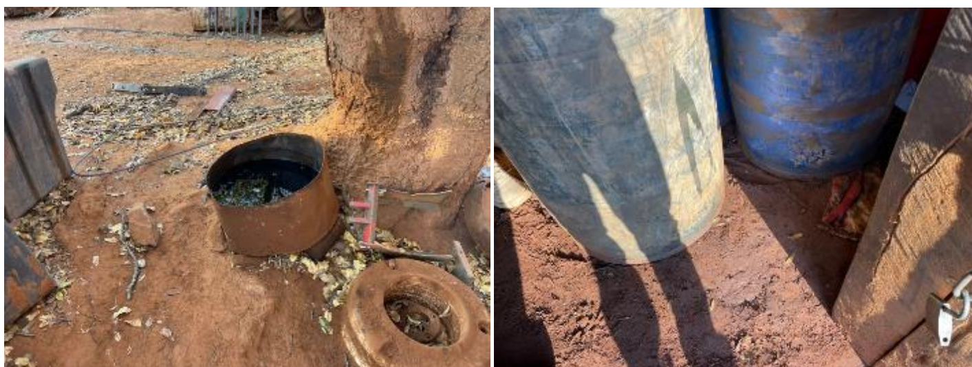
Figure 7 shows the Used oil not properly stored and the surface of the fuel storage facility that is not concreted
